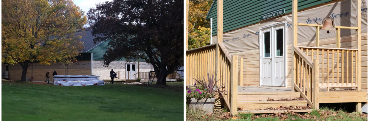
October 2026 - The Meadowmount Facilities team works to replace old siding on the exterior of Campe Concert Hall ahead of the coming winter.
